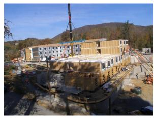
Hunter Modular Construction completed the erection of 129 modular units to form the 97,000 plus square feet permanent Residence Hall for ASU. HMC was contracted by Clayton and worked with JS Clark.
